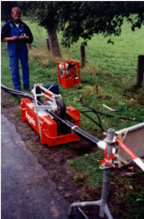
Laying of 3 x single core 30 kV
